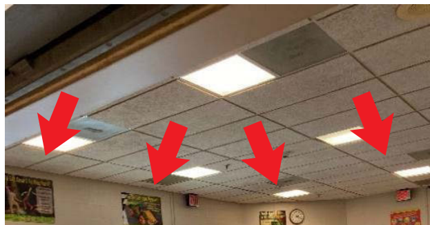
Bay Pines Center Cafeteria showing posters, near the ceiling
